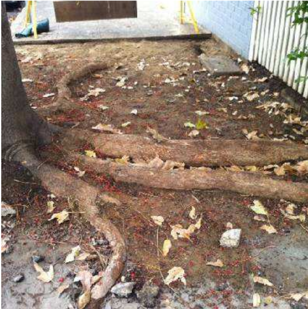
Figure 3. Example image of hand excavation, retaining and not damaging roots 30mm in dia or greater - prior to install of Filtapave © around existing tree (source: Sustainable, Lightweight Filtapave Manufacturers | Sydney )
