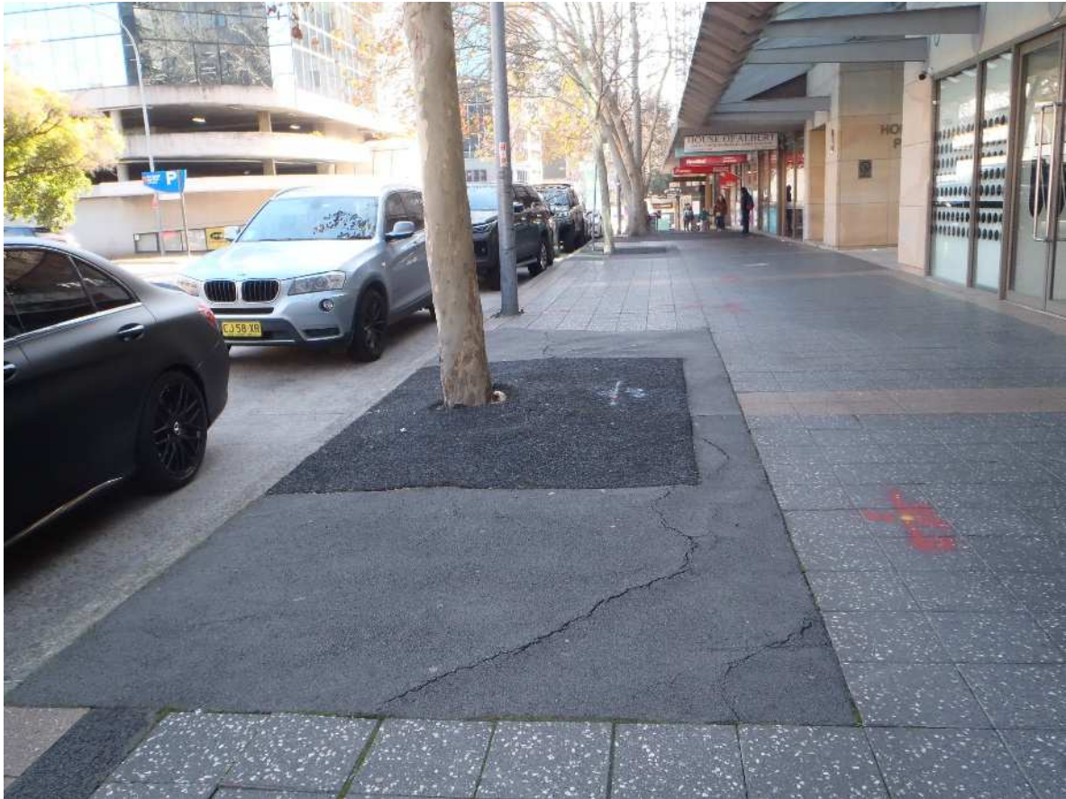
Figure 11. Base condition of T10 . Proposed for retention. Surface cracking in asphalt visible. Date: 8 August, 2023. Source: ELKE
