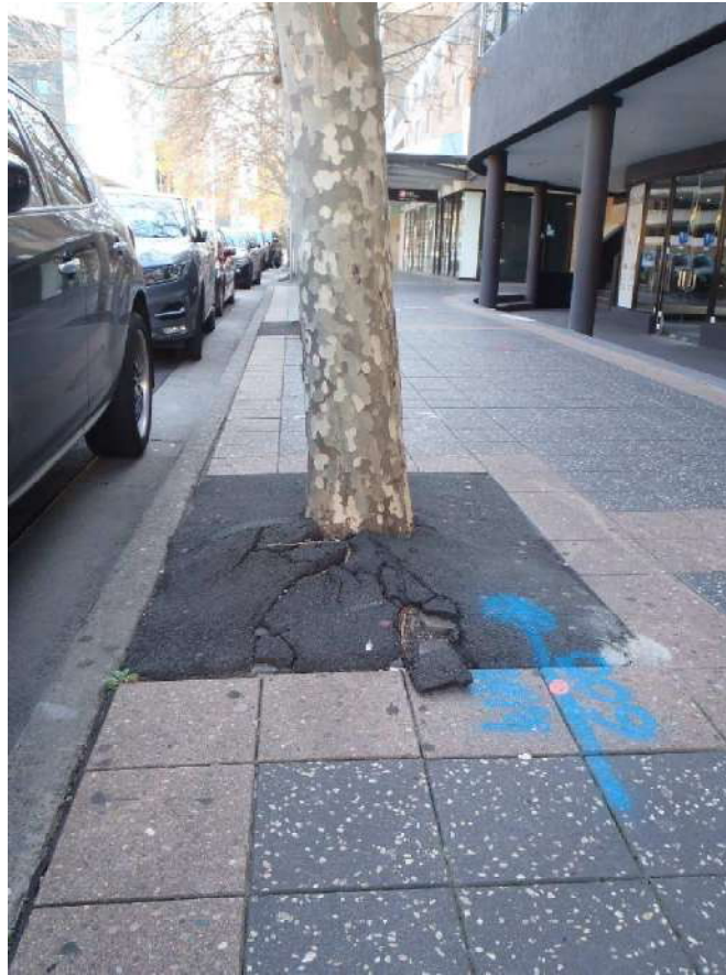
Figure 15. Photos showing T12 and T13 proposed for retention. Photo at the bottom shows displacement of asphalt indicating root zone upheaval indicating inadequate soil volume. Date: 8 August, 2023. Source: ELKE
