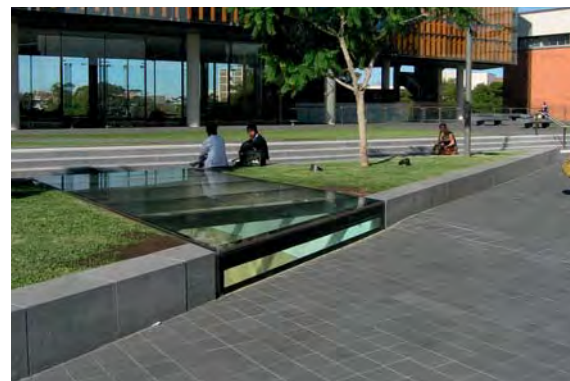
University of Sydney - Skylights
