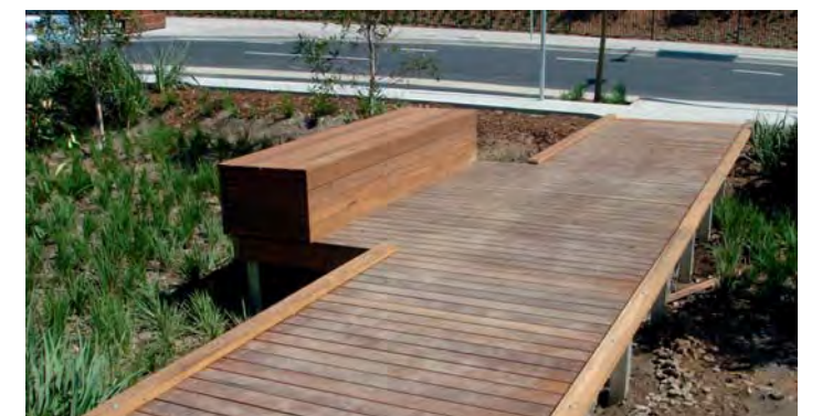
Rouse Hill - Timber Crossing
