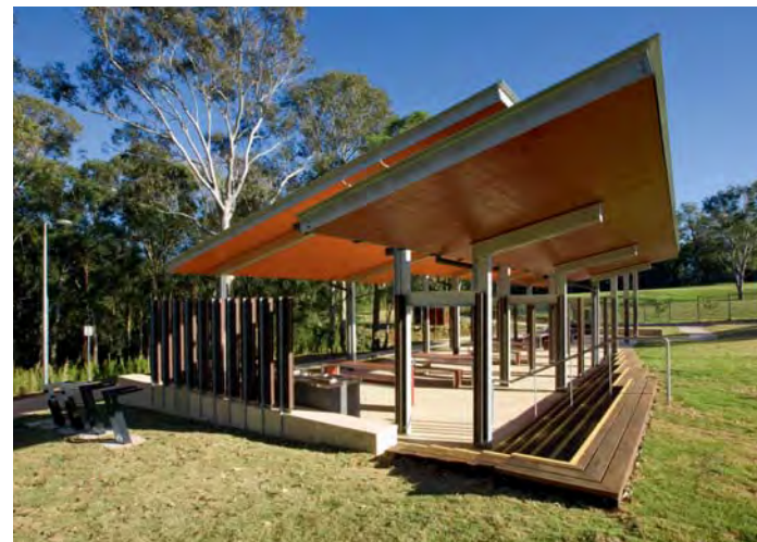
Rouse Hill - Shade structure
