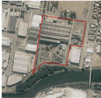
Figure 25 1980s aerial view with subject site outlined in red.
