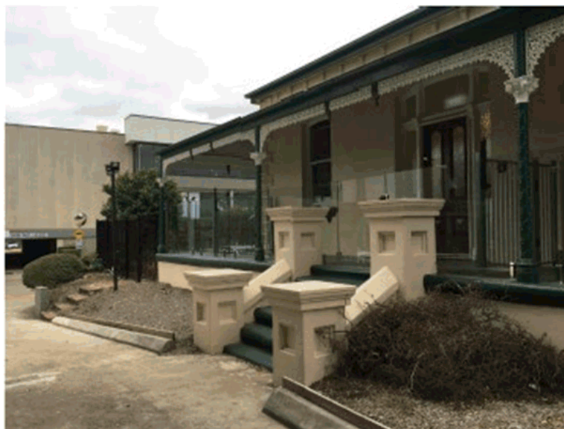
Figure 3 – Truganini House, western frontage (Source: Urbis)
