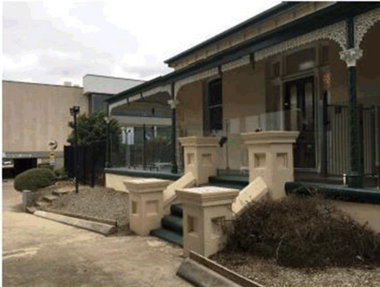
Figure 2: Truganini House (western frontage)
