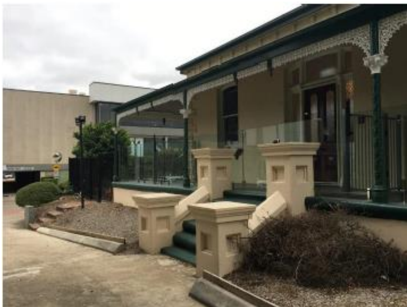
Figure 2: Truganini House (western frontage)
