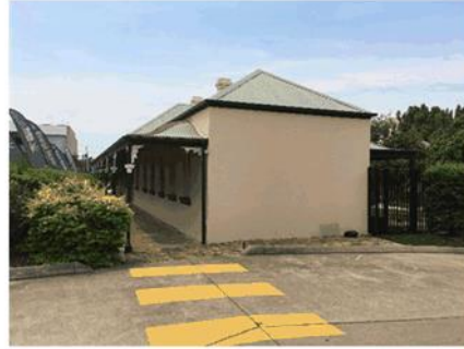
Figure 8 View of the western wing of the house, referred to as the barracks and the stables
