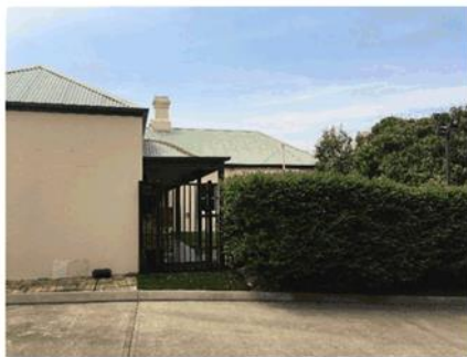
Figure 9 Western side of Truganini House defined by kerbs and hedging. There is a landscaped yard to the southwest of the house, which is used by the childcare centre
