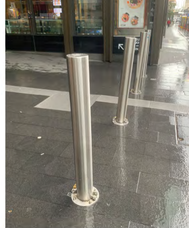
Stainless steel bollards
