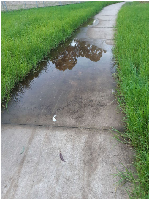
Figure 5 - Image showing pooling on pathway
