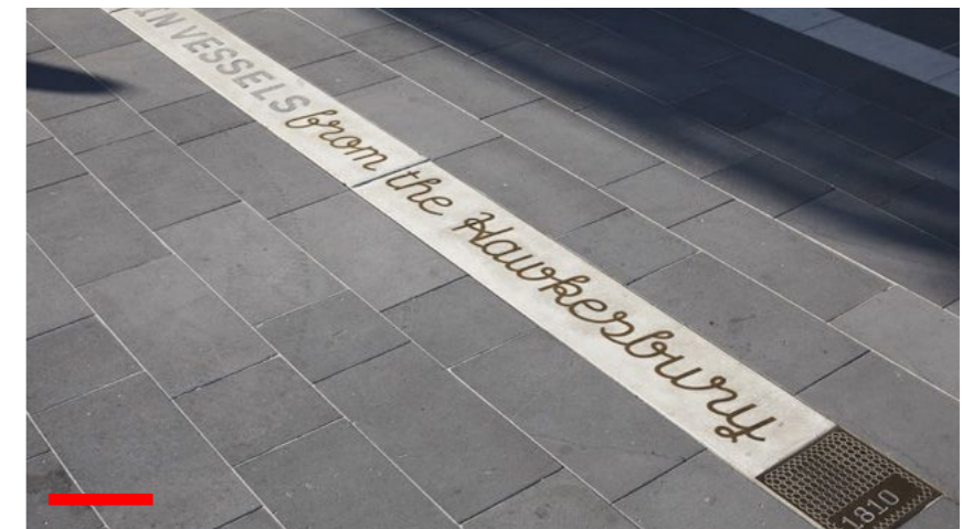
3. INTERPRETATIVE INLAYS Metal inlays to be used as wayfinding of creek alignment
