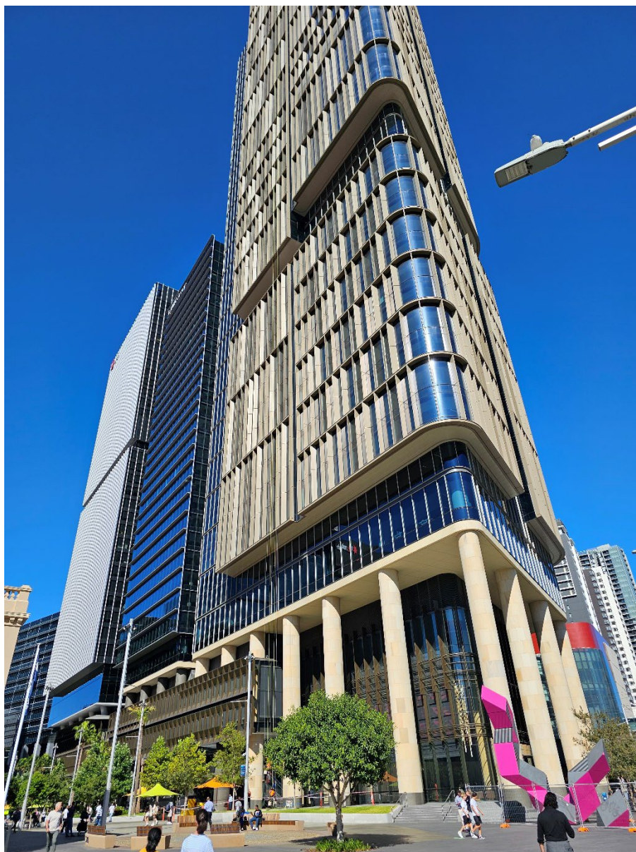
Figure 2 – Recently completed commercial office towers on Walker Corporation Landholdings at Parramatta Square, which is subject to rezoning under this planning proposal (known as 4 & 6 & 8 Parramatta Square).
