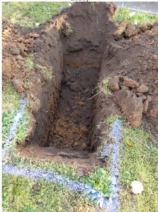
Photograph 8: View of the material from natural material from TP1(25 May 2023).
