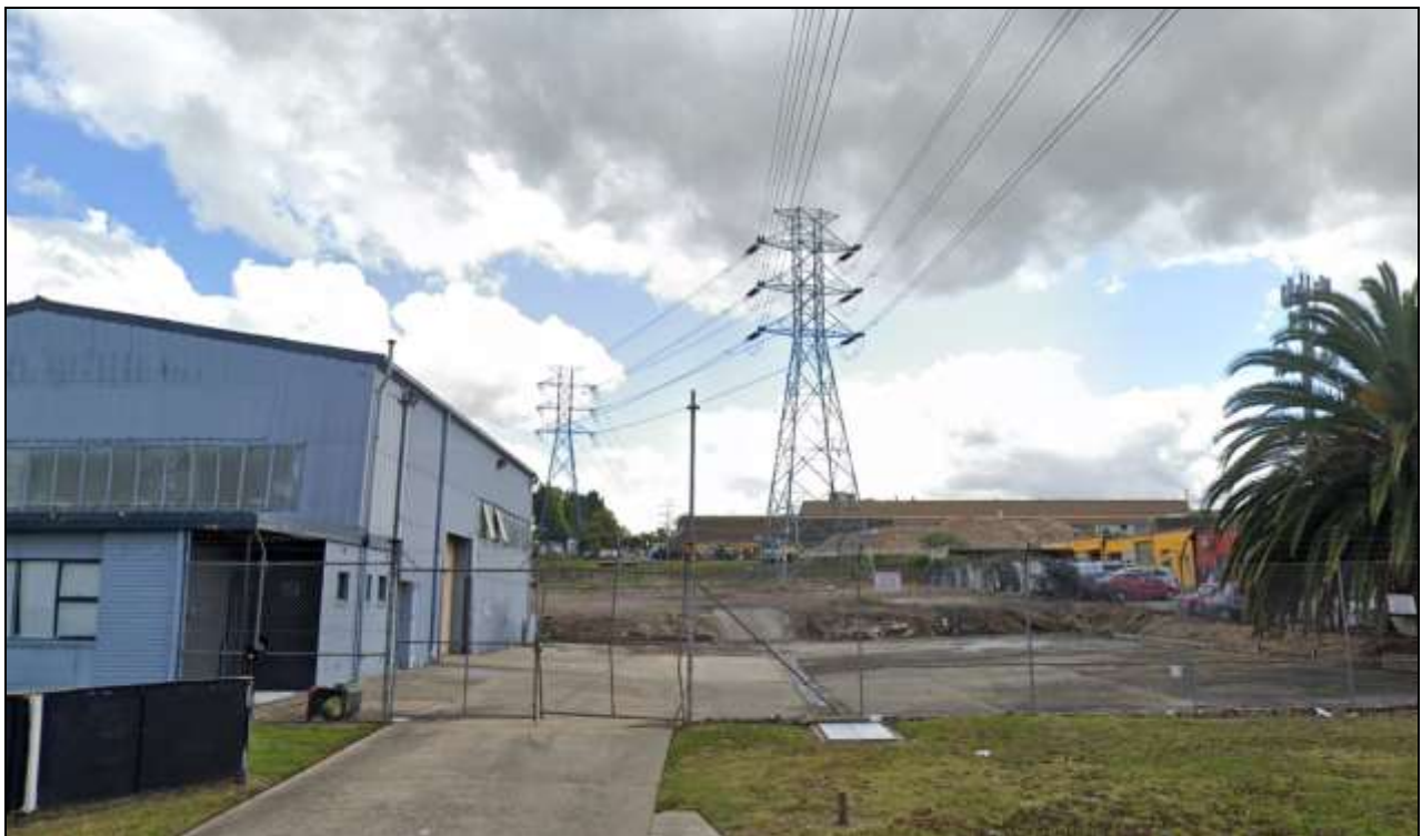
Figure 7 – HV Transmission in the Site (source: Google Maps)
