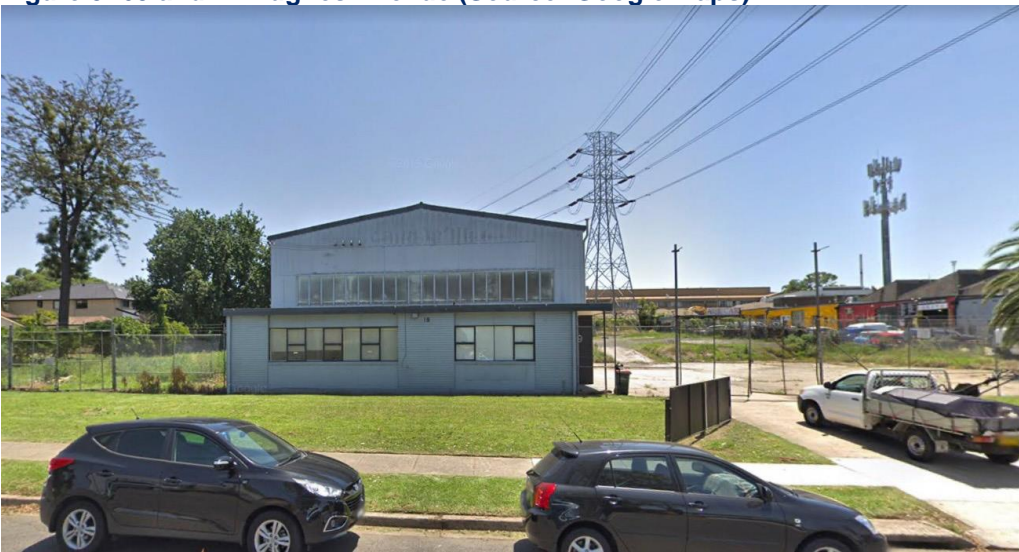
Figure 6: Former Tomola Motors site (now vacant) and high voltage powerline at 19 Hope Street (Source: Google Maps)
