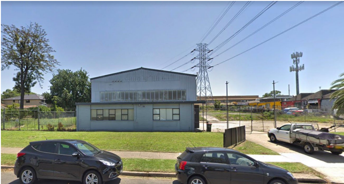
Figure 3: Former Tomola Motors Site at 19 Hope Street (Source: Google)
