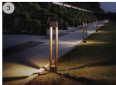
Lighting to pathways
