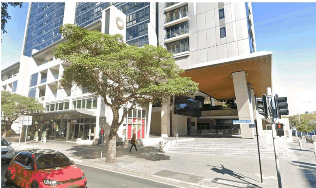
Figure 10 – Street view of the subject site from Marsden Street, Parramatta
