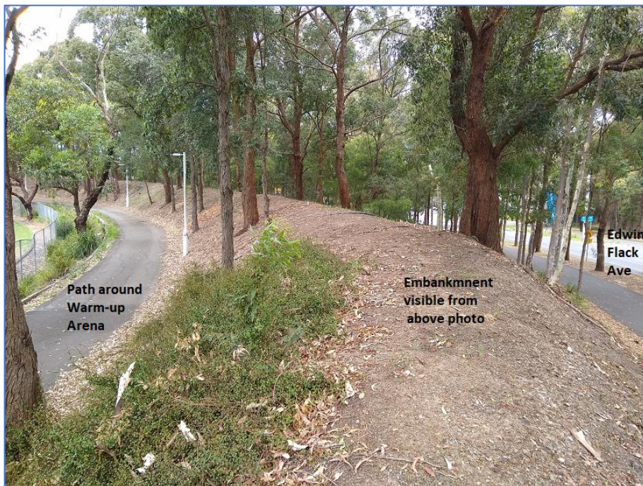
Embankment between wider path alongside NE side of Edwin Flack Ave and path around the Warm-Up Arena.
