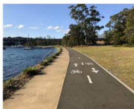
Separated cycleway in park
