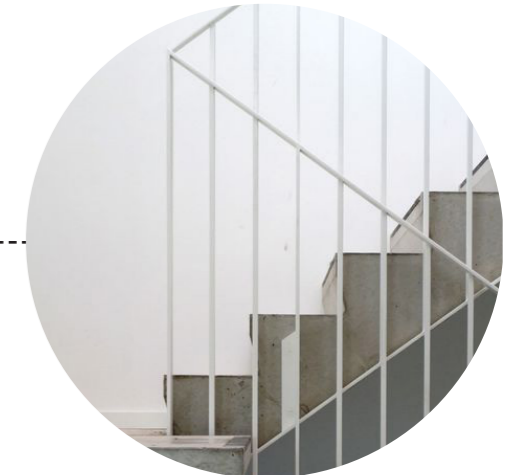
Steel Rod and Flat Balustrade
