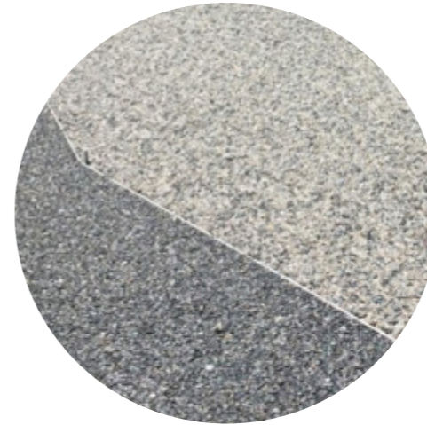
Viewing Platform Paving Open-pore Resin Bound Aggregate
