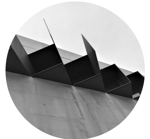
High Level Screens Steel Plate with Expanded Metal infill. Recoatable Paint Finish
