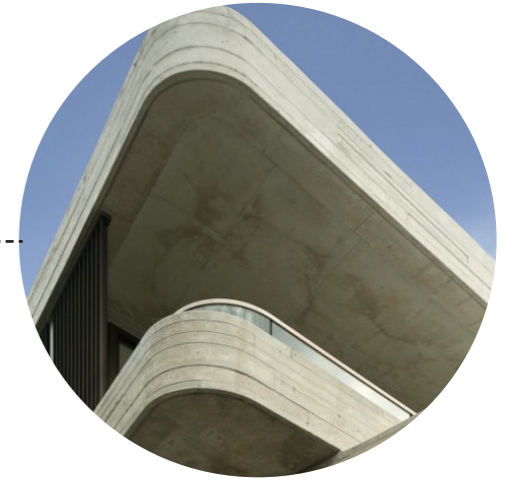
Off-Form Concrete Awning
