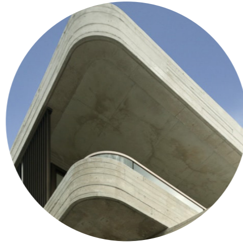
Lower Awning Off-Form Concrete - Robust and easy to maintain.
