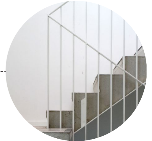
Steel Flat and Rod Balustrade
