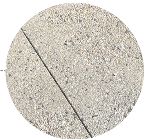
Washed Aggregate Concrete Slab
