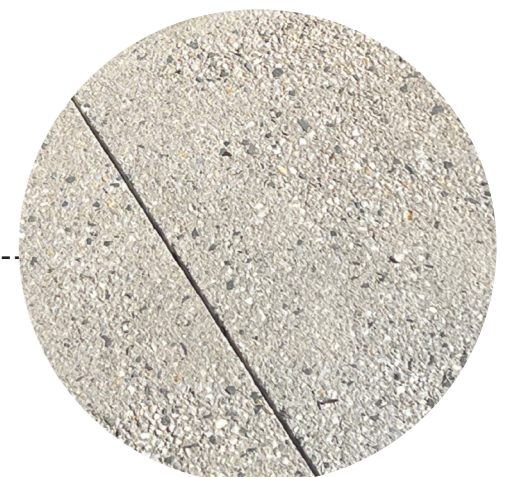
Washed Aggregate Concrete Slab
