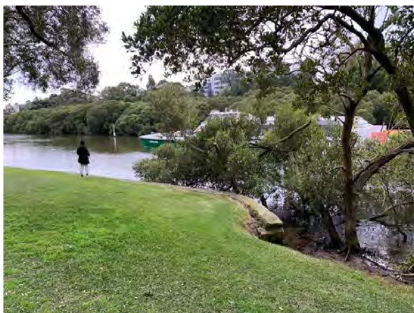
Figure 34 Sandstone walling associated with the Wharf. Facing north-west.
