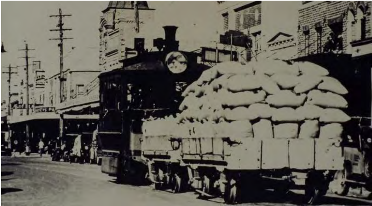
Figure 16. c.1940 photograph of tram along the George Street tramway. Source: City of Parramatta Council's Research and Collection Services. Object number LSP01059.
