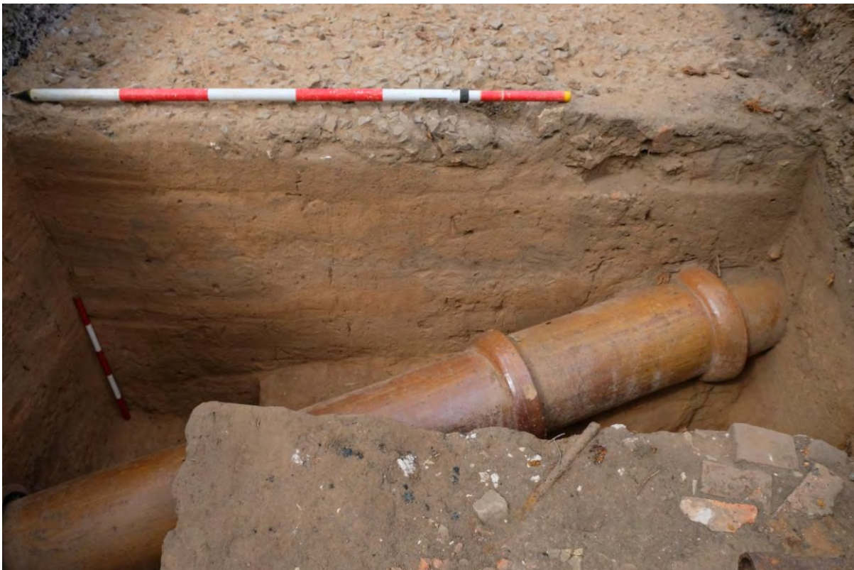
Figure 46. ATP5 within TT5. Excavation of PSB around service trench.
