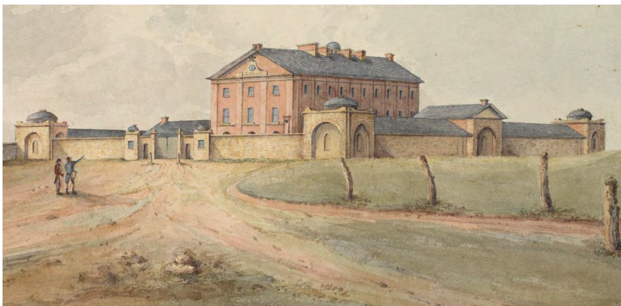
Figure 59. Hyde Park Barracks c.1820. Source: SLNSW FL3323021
