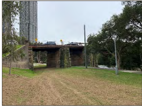
Figure 25 Disturbance associated with Gasworks Bridge.
