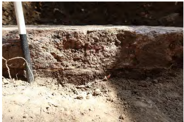
Figure 57. Northern face of bricks associated with gasworks structure 10.004 and detail of damage caused by demolition works, facing south.
