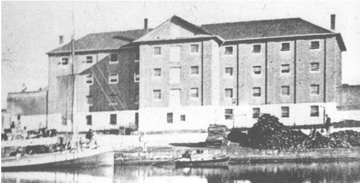
Figure 11. c.1870 photographic plate showing the former Commissariat Store/Lower Military Barrack, now in use as the Parramatta Benevolent Asylum. Source: Shylie & Ken Brown, Parramatta: a town caught in time, 1870 , Hale & Iremonger, Sydney.1995
