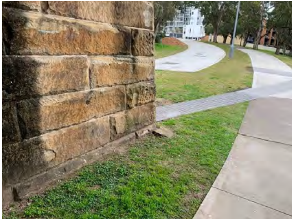
Figure 36 Sandstone piece underneath Gasworks Bridge. Facing west.
