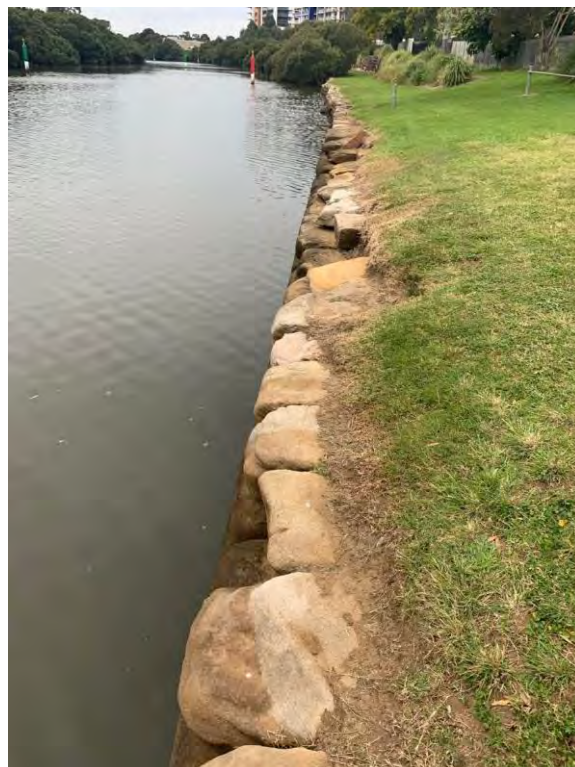
Figure 33 Example of sandstone wall along the Parramatta River.
