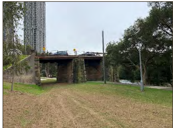
Figure 39 Disturbance associated with Gasworks Bridge underpass.
