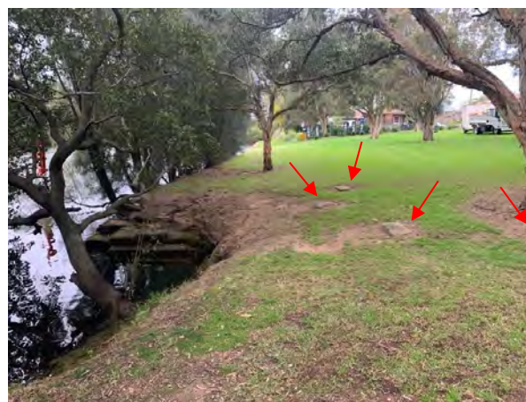
Figure 35 Sandstone walling associated with the Wharf. Additional pieces of sandstone marked with red arrows. Facing east.
