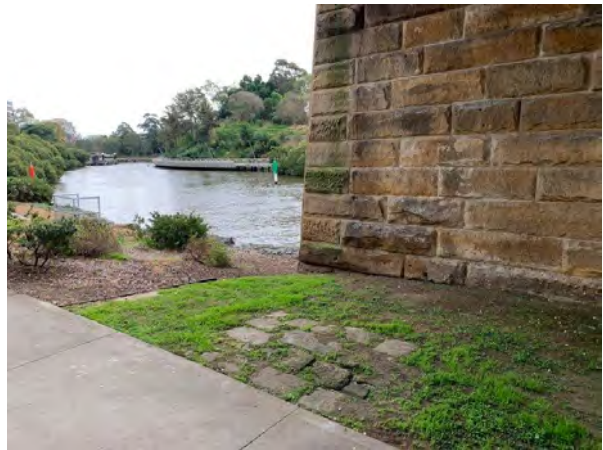
Figure 37 Sandstone flagging underneath Gasworks Bridge. Facing west.
