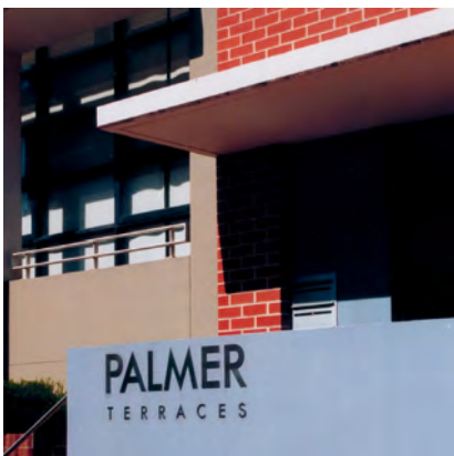
Signage gives identity to the building entry and provides legibility for visitors.
