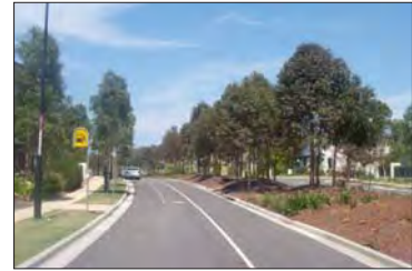
Asphalt roadway, Newington
