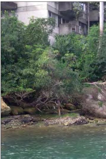
Examples: Retention / reestablishment of sections of natural foreshore junctions incorporating riparian vegetation is the optimum outcome in terms of habitat values
