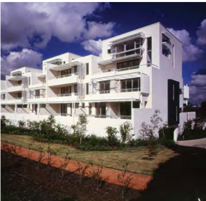
Sun shading is an integral component of the building form and facade design.
