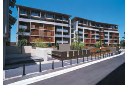
This facade has a strong balance of horizontal and vertical framing elements with sunscreen and balustrade infill components
