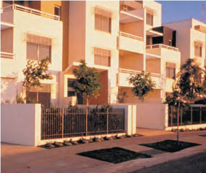
A picket and pillar fence defines the street boundary, clearly demarcating 'public' and 'private' space.
