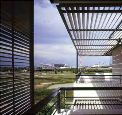
A combination of louvres provides shading for different times of the day.
