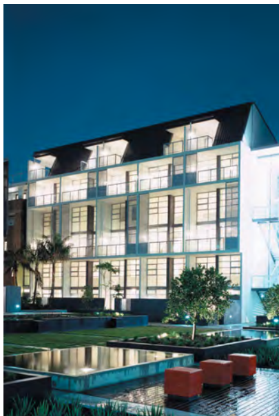
This modern version of the attic contributes to a dynamic and vibrant roofscape at night time.
