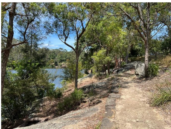
Figure 13: View of existing sandstone pathway edging within proposed construction access track
