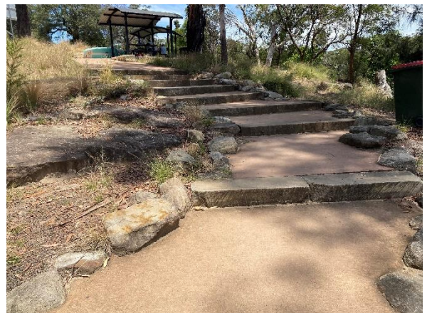
Figure 3-28: View south-west showing concrete steps leading towards the carpark
