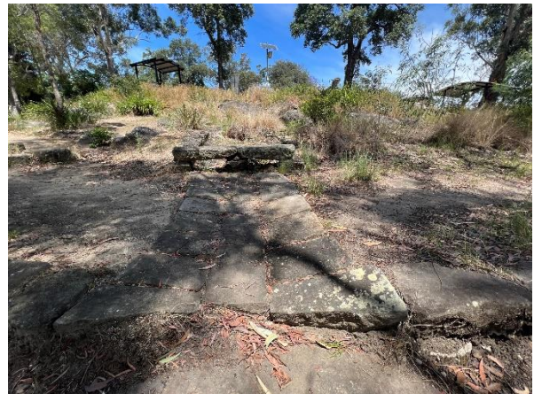
Figure 12: View of existing sandstone culvert structure within proposed construction access track
