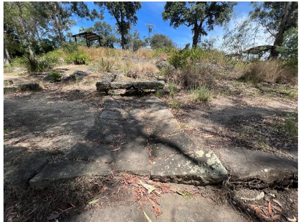
Figure 3-34: View of existing sandstone culvert structure within proposed construction access track
