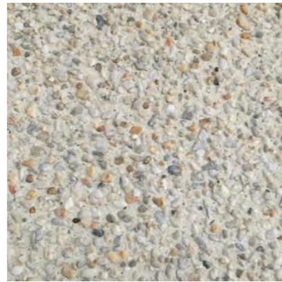
EXPOSED AGGREGATE CONCRETE PAVING Throughout proposed works
