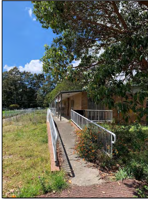
Photograph 10: View of the western end of the existing amenities building that is to be extended at its eastern end.
