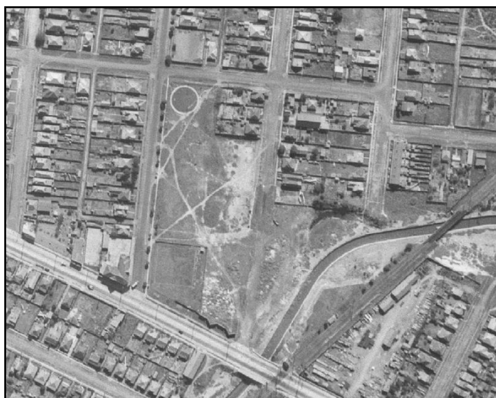
Figure 6.1 – 1943 Aerial Photograph of FS Garside Park
