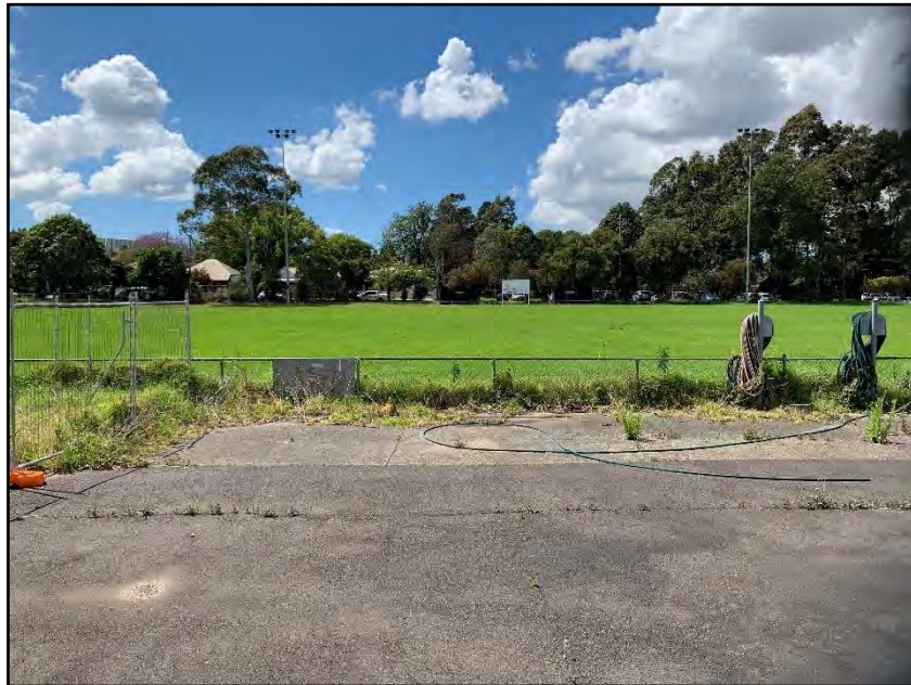
Photograph 11: View of the existing playing field looking east towards Onslow Street.
