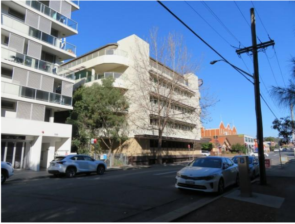
Figure 6.16 The site looking south from Wigram Street.
