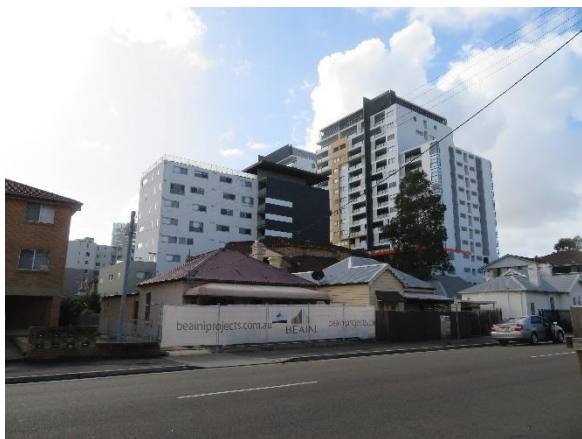
Figure 5.10 Marion Street—northern side with heritage items in the foreground.
