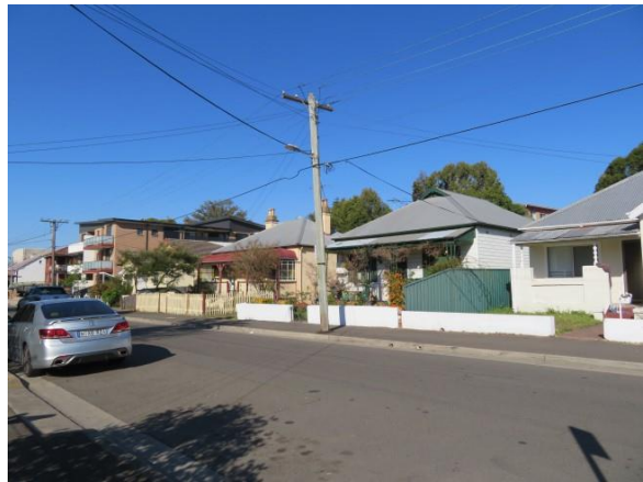
Figure 5.19 Dixon Street—outside the conservation area.
