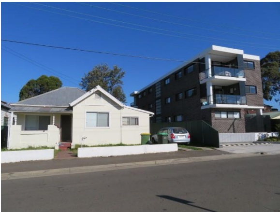
Figure 5.18 Dixon Street—outside the conservation area.
