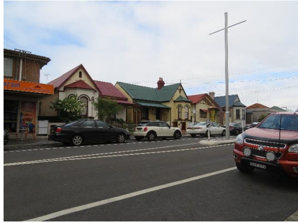
Figure 4.15 Heritage items and Harris Park Conservation Area at the southern edge of the South-East Interface Area.
