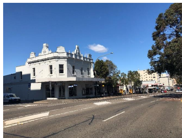
Figure 3.5 Church Street near Fennell Street, looking south.
