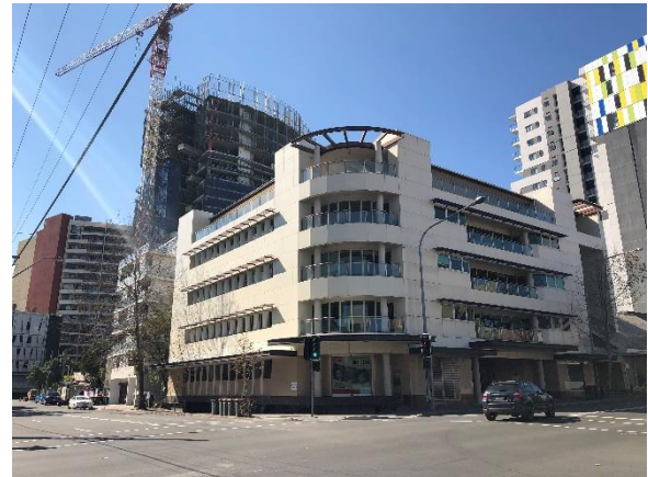
Figure 6.15 The site looking northwest.
