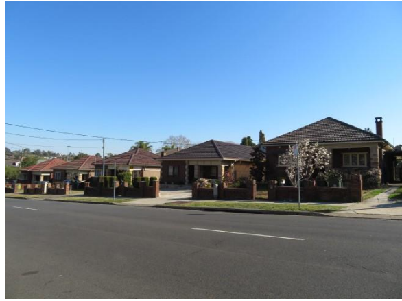
Figure 5.15 Marsden Street, western side—South Parramatta Conservation Area.
