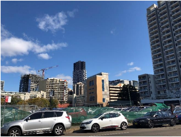
Figure 4.2 Northern Part of the SE Interface Area.
