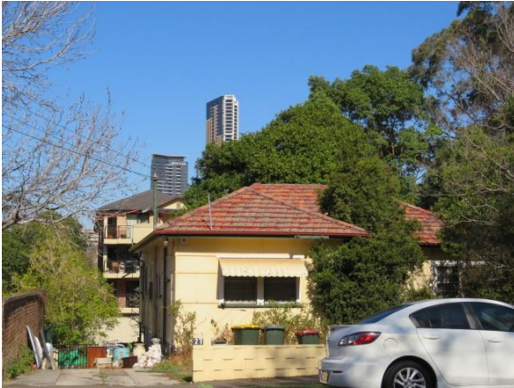
Figure 6.4 Existing cottage on the site.
