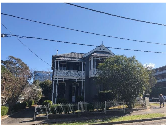
Figure 3.18 Sorrell Street Heritage Conservation Area—No. 53 Sorrell Street.
