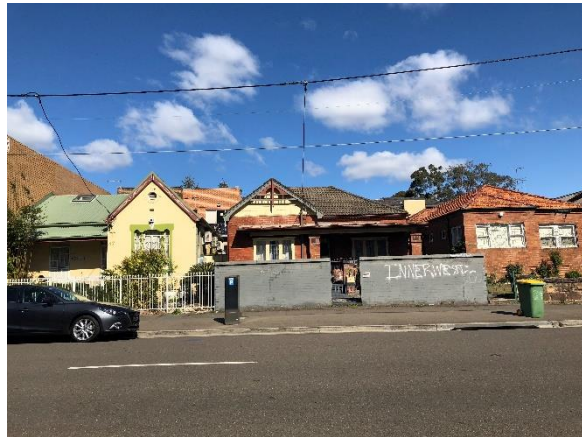
Figure 6.19 Heritage item at 37 Marion Street—approved to be demolished.
