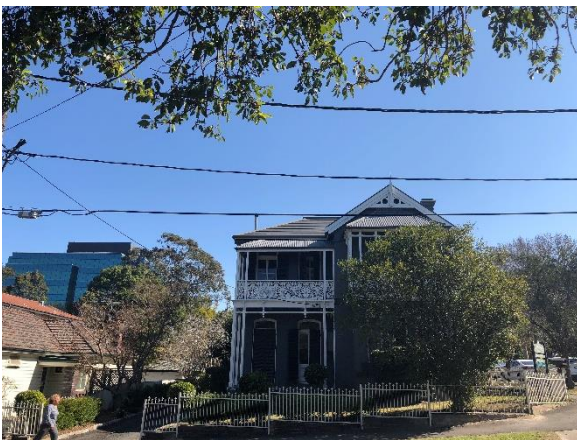
Figure 6.6 Heritage item at 53 Sorrell Street.
