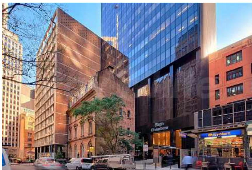
Figure 32: Sometimes a setback can be of benefit in providing a setting for a historic building within a CBD context (Source: Ray White Real Estate listing for 25 Bligh Street, Sydney 11 )
