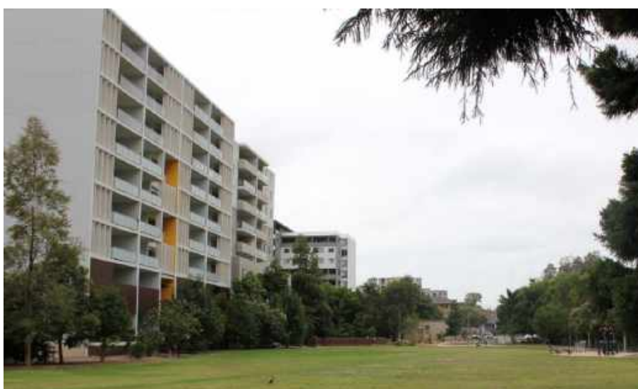
Figure 87: Apartments overlooking Jubilee Park, but with no connection to the place. (Source: HAA)
