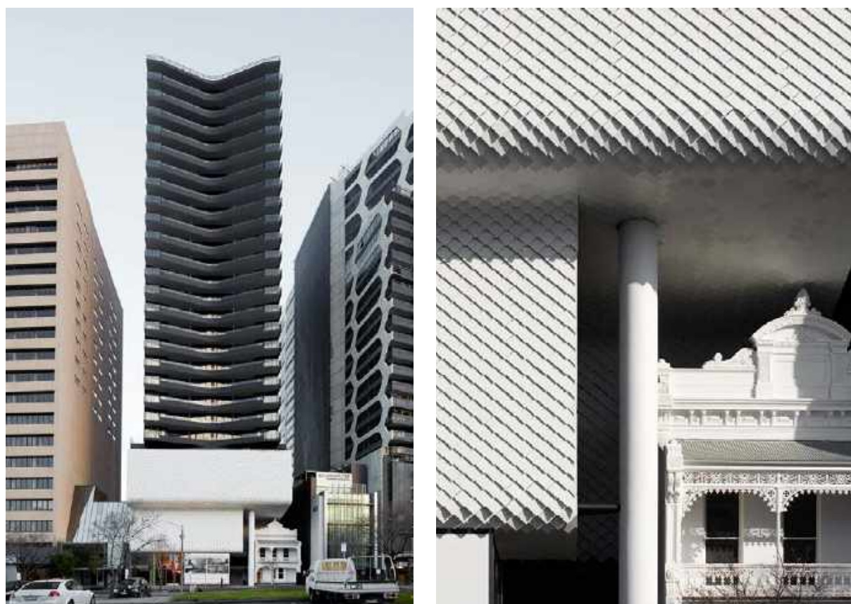
Figure 13: 50 Albert Road, South Melbourne – tower overhanging terrace house. An example of sidelining and swamping heritage, the impact of which extends across the city
