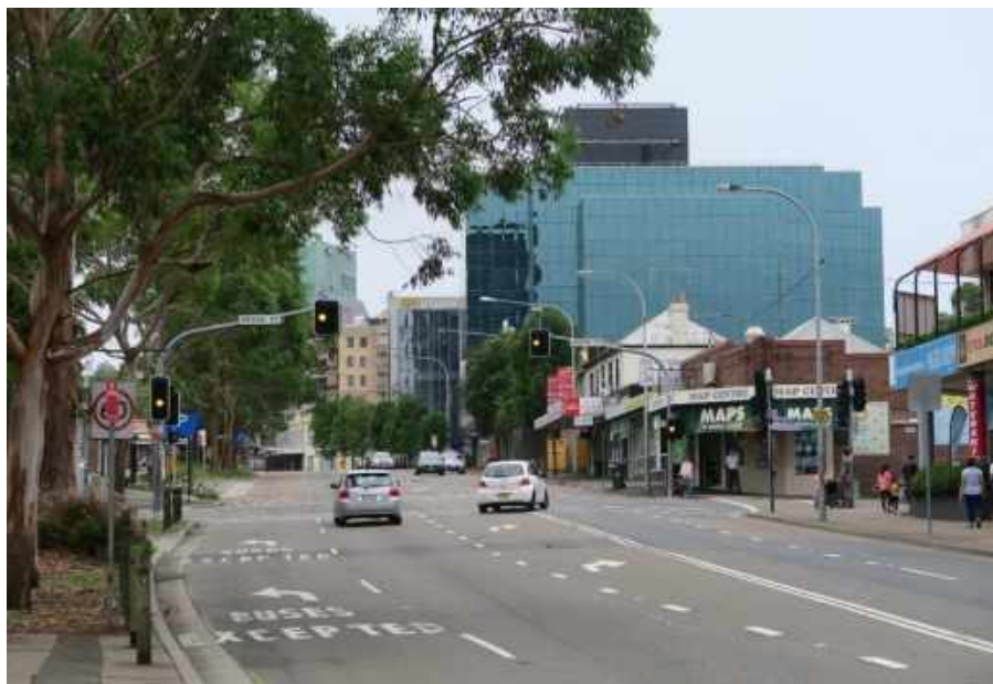
Figure 46: Church Street North (Source: HAA)
