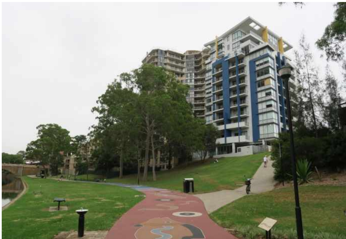
Figure 58: Parramatta River bank looking north (Source: HAA)
