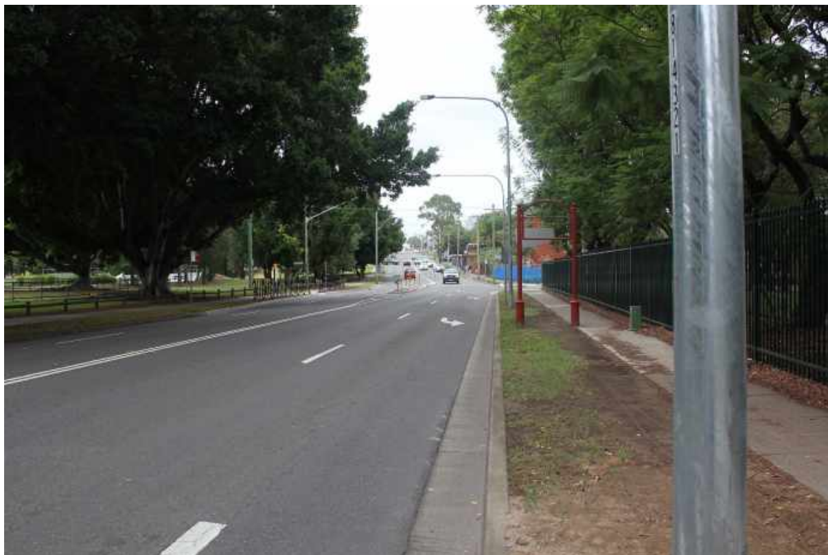
Figure 73: Harris Street looking south (Source: HAA)
