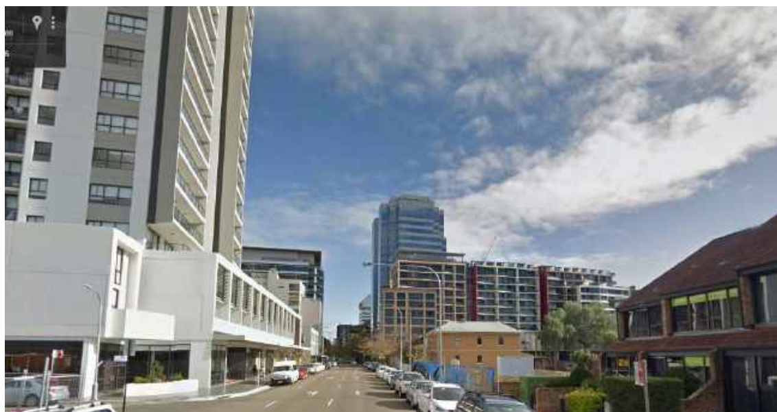
Figure 71: Podium showing amalgamation of lots in George Street, Parramatta and the early house Harrisford
