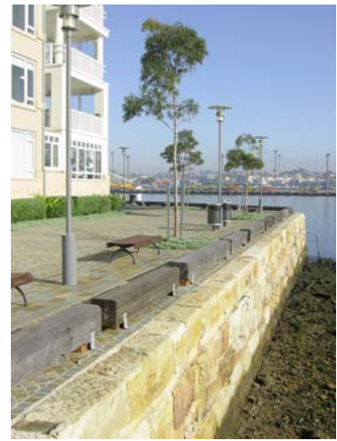
Pymont Waterfront: The foreshore promenade is to be the focal public domain space of Homebush Bay West - providing a place for activity, rest, and viewing
