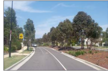
Asphalt roadway, Newington
