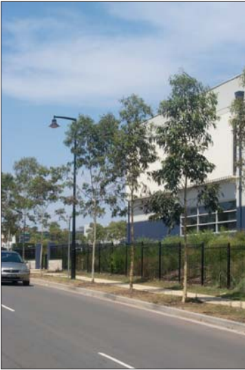
Concrete kerb and gutter
