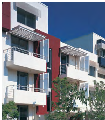
The detailed design of these partially solid balustrades, sun shades and privacy screens contribute to the overall facade composition of the building.
