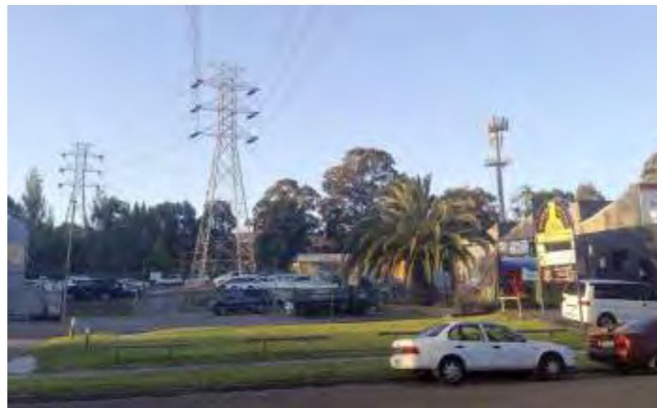
View 5 - Looking north from Hope Street at existing industrial around The Site and the high voltage power lines running along the western end of the Site.
