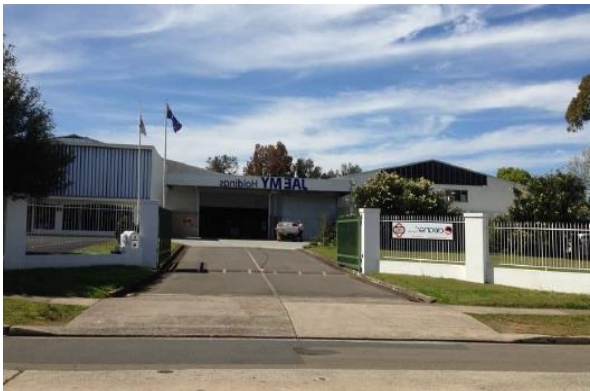
Figure 7. Existing building at 8 Wharf Road
