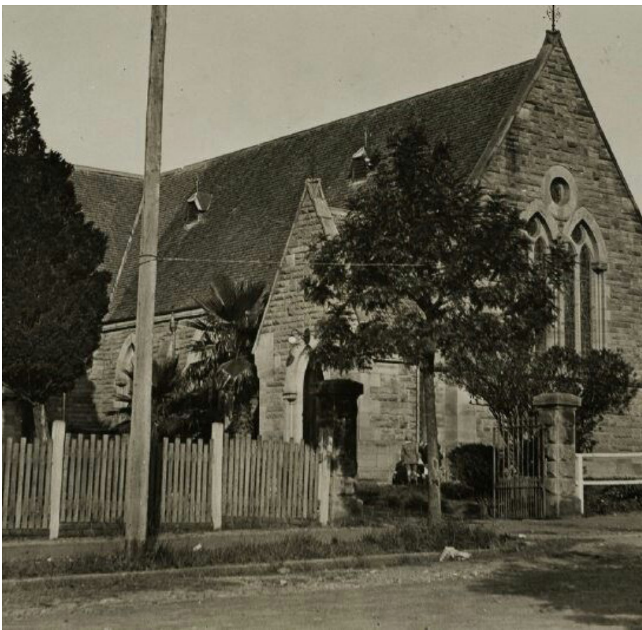
Image 7: St Mark's Anglican Church, built 1882.
