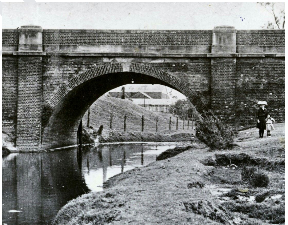
Image 1: Duck Creek Bridge, Granville is the first and/or the oldest surviving brick semi-circular arched bridge to be constructed in Australia.
