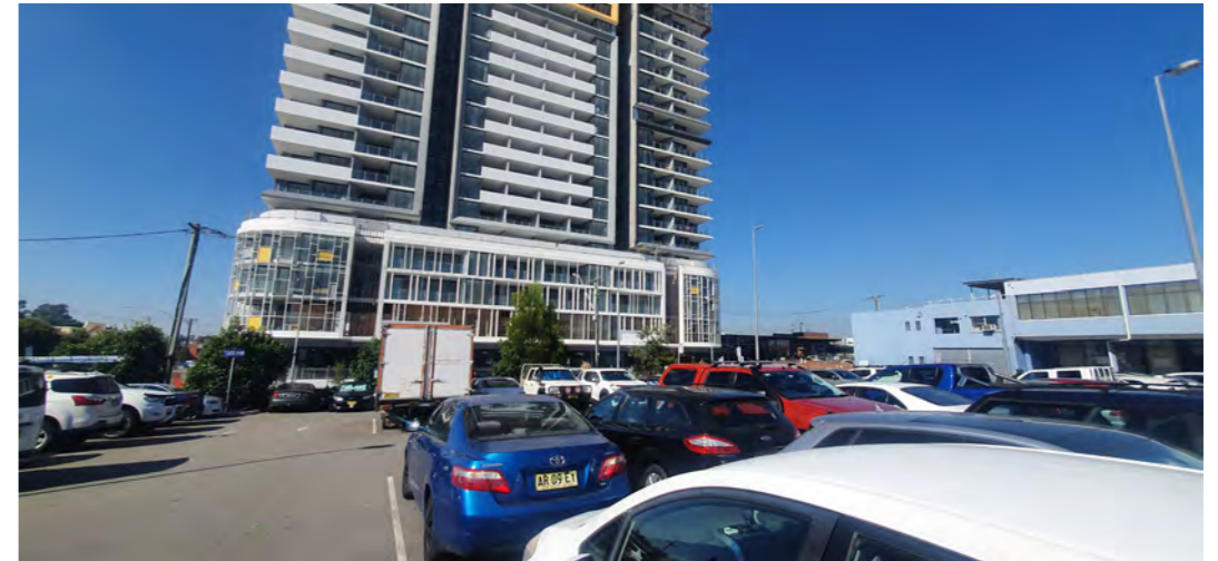
Residential apartments under construction directly adjacent to site.
