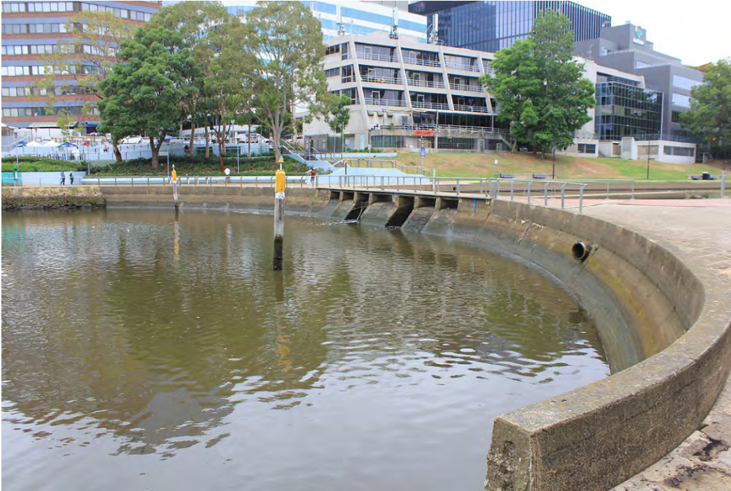
Figure 4-7 Looking south west across the Charles Street weir. (Curio, 2019)
