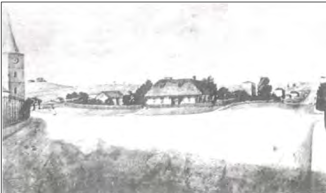
Figure 3.2: Sketch of the Native Institution Site/Buildings. Dated To c.1820 (?) (Source: Royal Australian Historical Society Glass Slide 4636, Reproduced In Kass, Liston & Mccllymont 1996: 105.)
