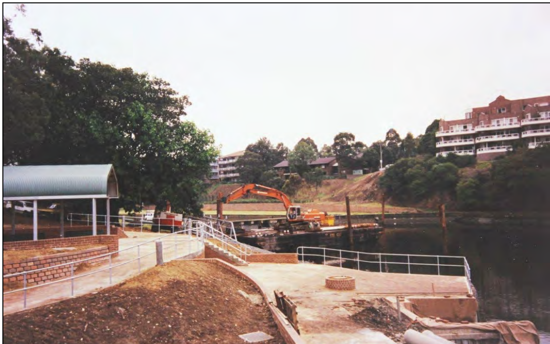
Figure 3.13: 1988 Construction of Charles St Ferry Wharf
