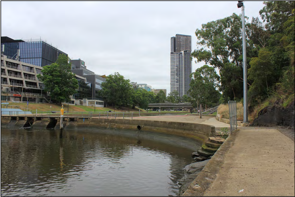
Figure 6.4: Charles St Weir, View west (Source: Curio 2019)
