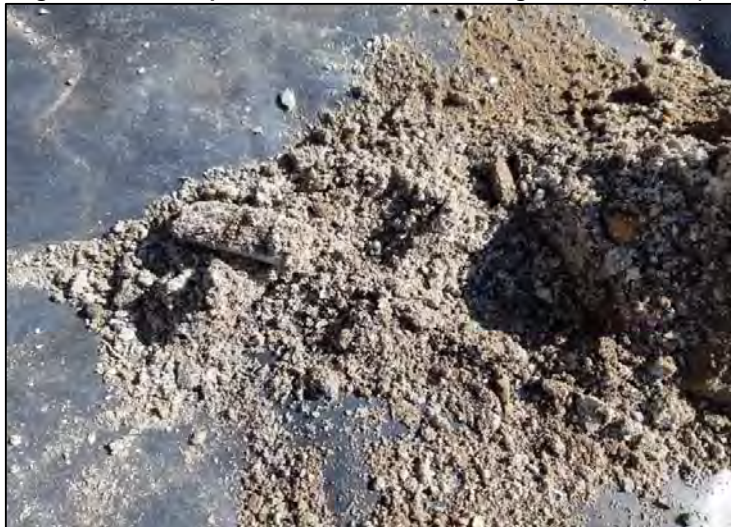
Image 8.5.1 View of potential asbestos containing materials (ACM) as observed in BH06
