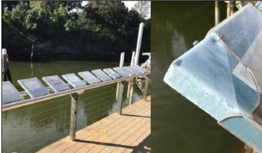
Figure 28: Handrail art panels (Source: Extrablack via SMM)
