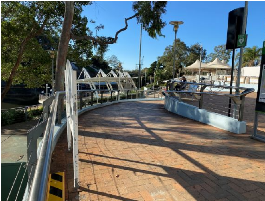
Photo 2: Mid level view looking east along pedestrian ramp
