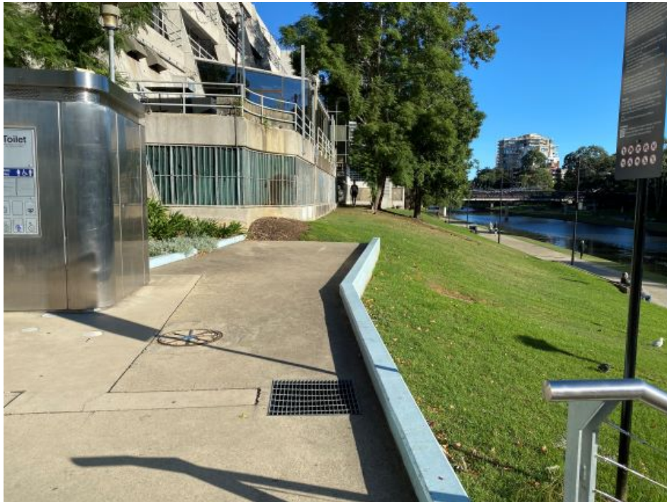
Photo 10: View west showing 94 Phillip Street commercial building with basement car parking
