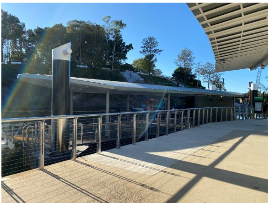
Photo 11: Parramatta ferry wharf, renewed in 2019
