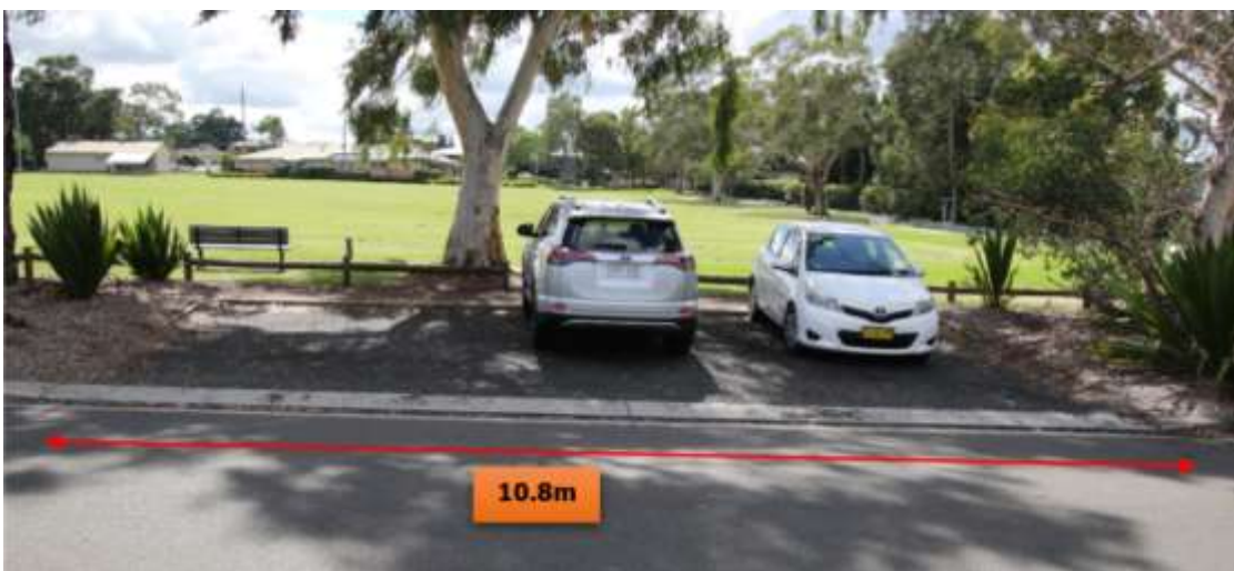
Photo 4.20: Location #13: 4 (four) off-street parking spaces (Photo: Traffic Engineering Centre Pty Ltd)
