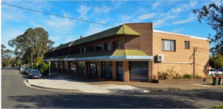
Figure 3 Looking west towards Bartlett Street Shops
