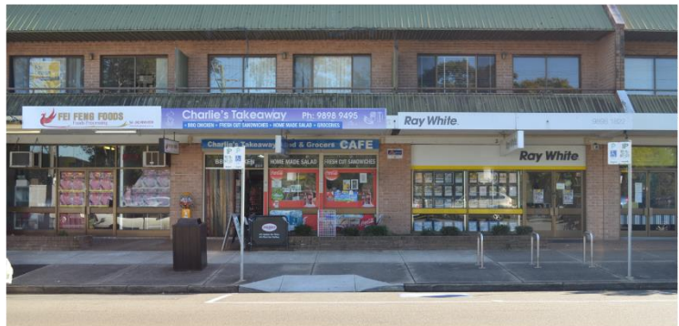
Figure 8 Looking northwest towards tenanted shopfronts at Bartlett Street Shops
