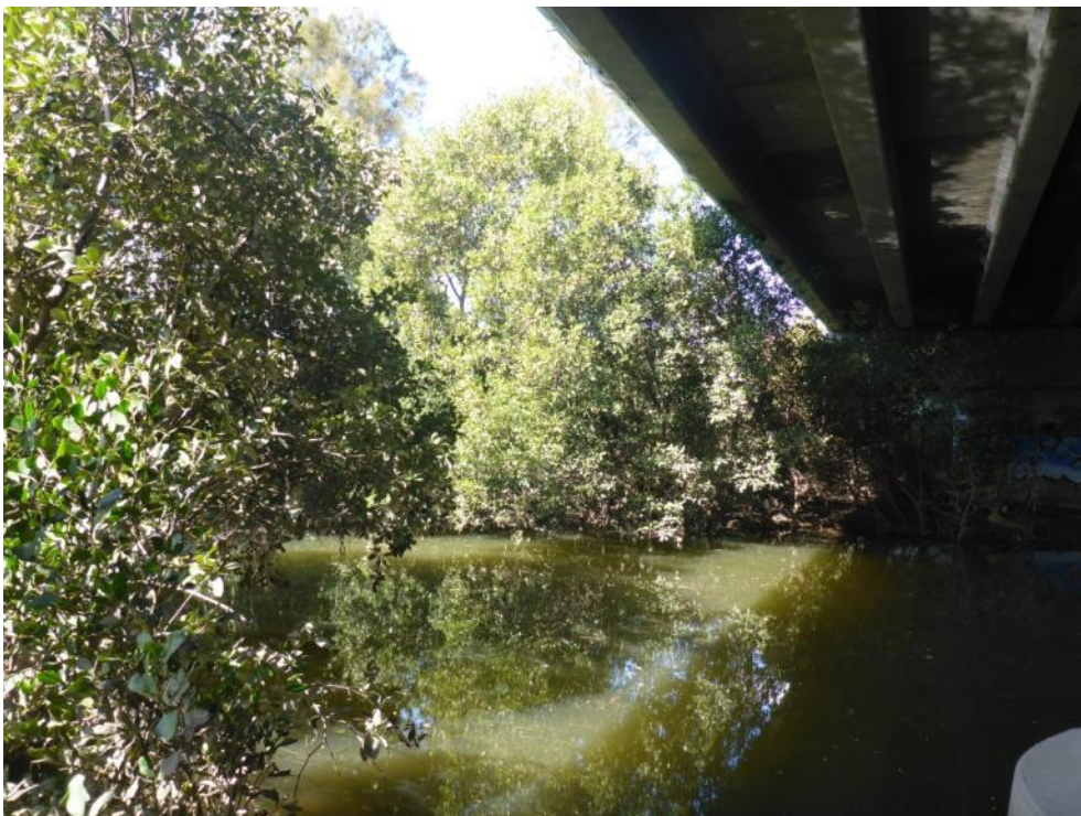
Photograph 3.12 Saltmarsh and mangrove communities shaded by the M5 Motorway at Salt Pan Creek (view northeast: 27/09/2017 at 15:09 hrs.)
