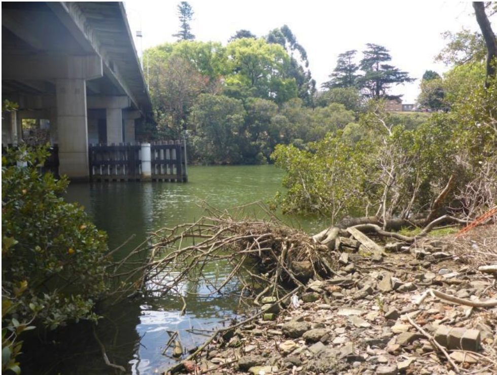
Photograph 3.3 Saltmarsh and mangrove shaded by James Ruse Drive over the Parramatta River (view northeast: 27/09/2017 at 13:35 hrs.)
