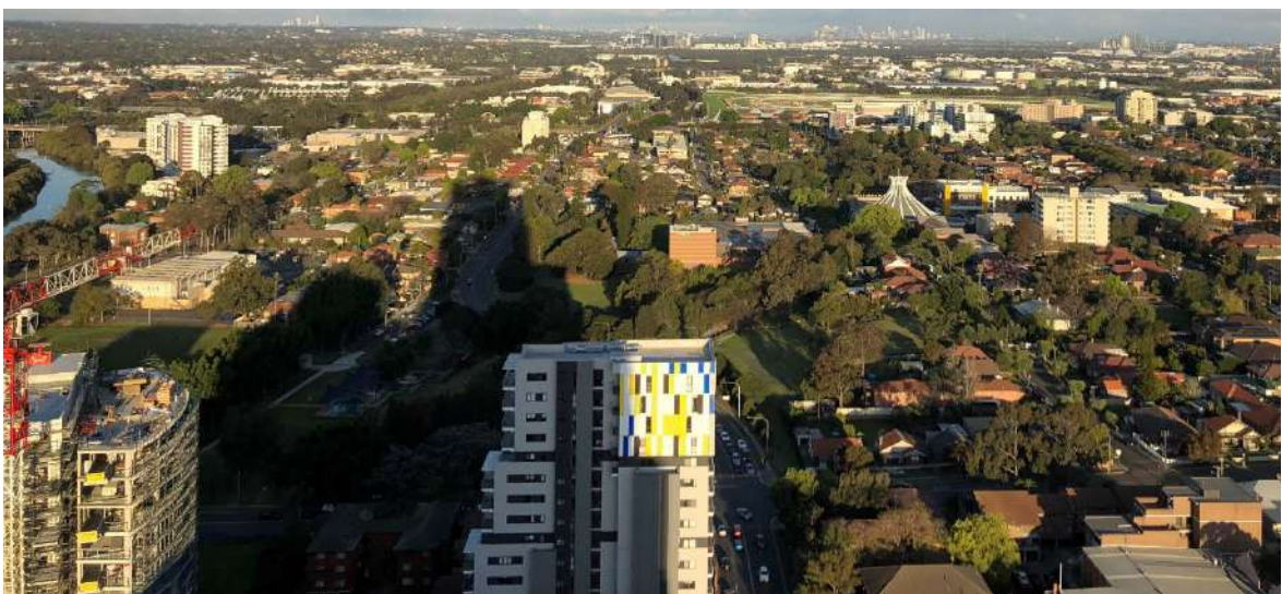
Figure 2 - Overshadowing cast by existing development in the Parramatta CBD. Photo taken from Level 33 at 11 Hassall Street, Parramatta, on 8 October 2018 at 6:15pm (UTC+11).
