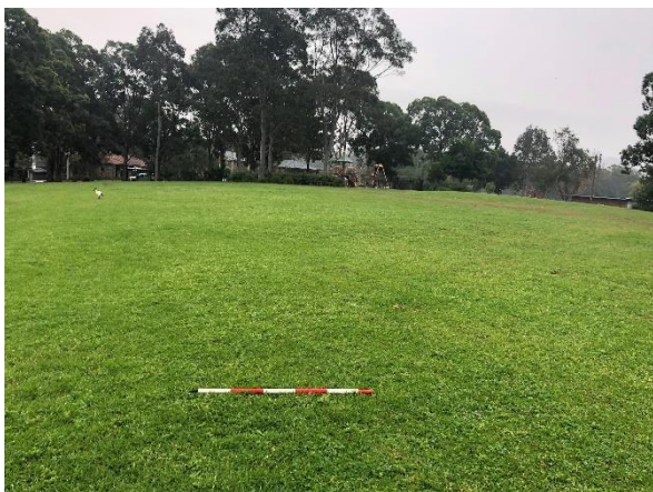
Figure 9: Rectangular slumping in the centre of the park
