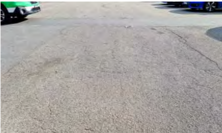
Photo 6.4 (Photo: Traffic Engineering Centre Pty Ltd)
