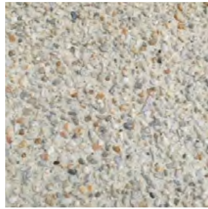
EXPOSED AGGREGATE CONCRETE PAVING Areas Surrounding Amenities Building
