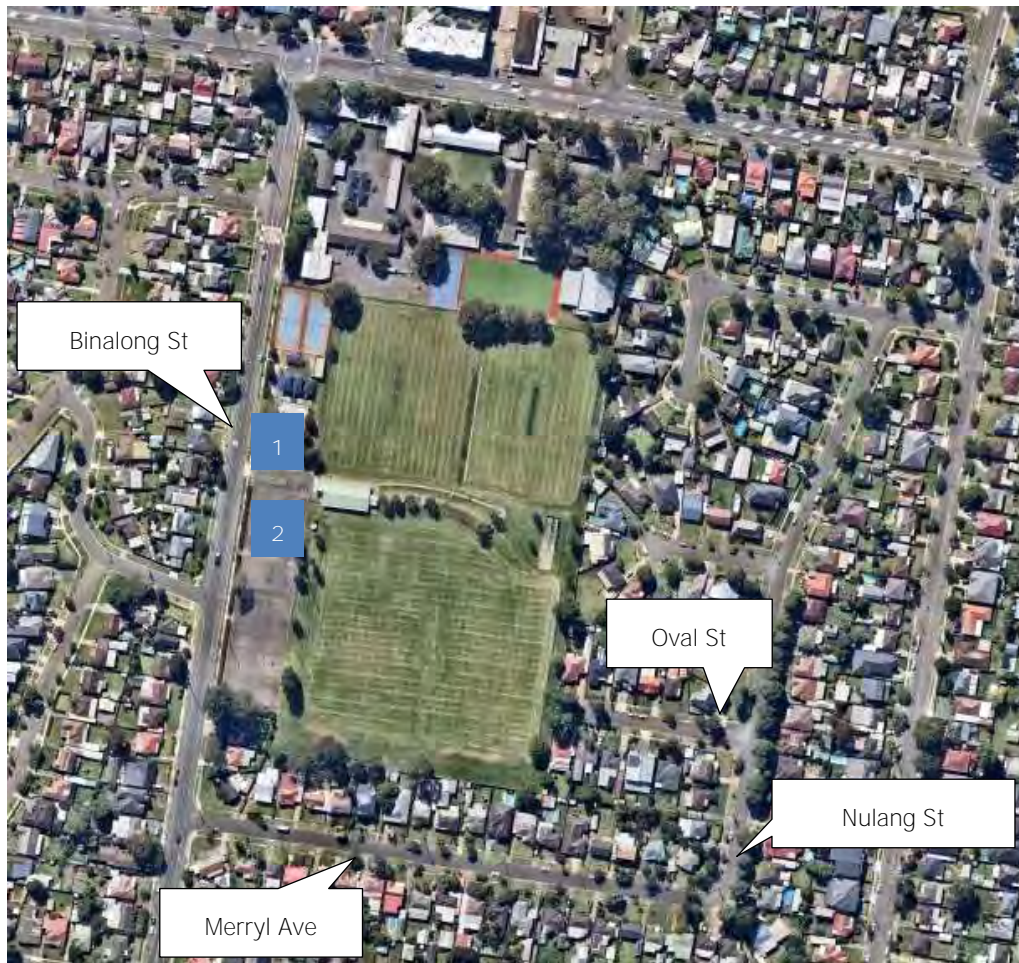
Figure 4.4: Locations of permanent off-street parking, adjacent to the Binalong Park (Source: Nearmap)
