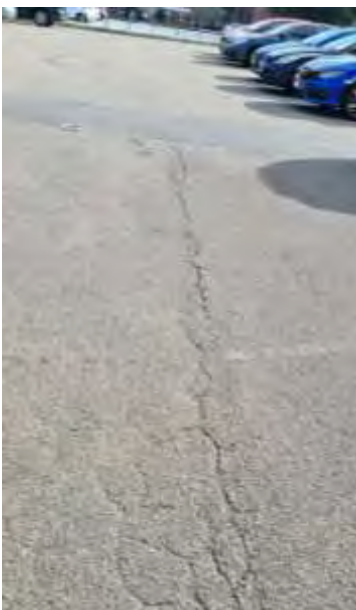
Photo 6.5 (Photo: Traffic Engineering Centre Pty Ltd)
