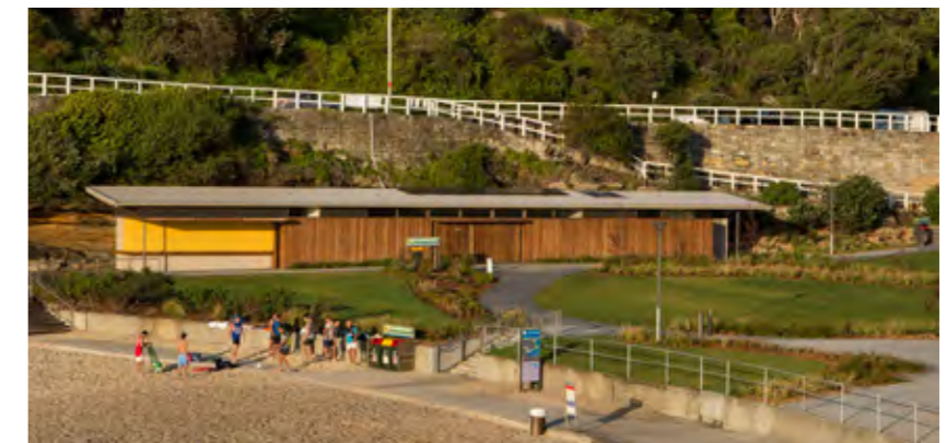
TAMARAMA KIOSK AND CHANGE ROOM Lahznimmo
