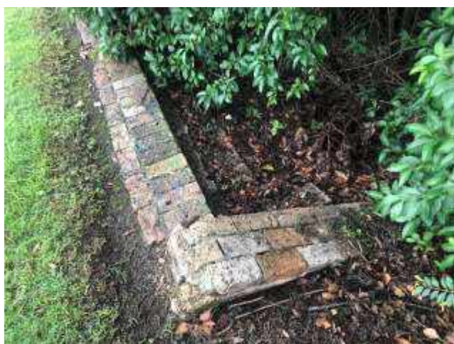
Plate 3.9. Brick staircase, view east.
