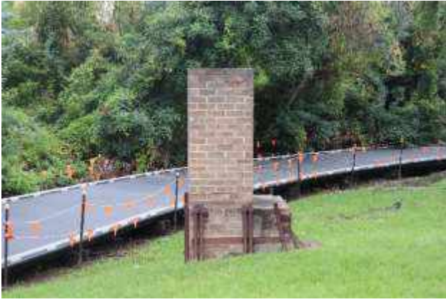
Plate 3.5. The brick incinerator, view south. Note the slightly raised pathway to the background.
