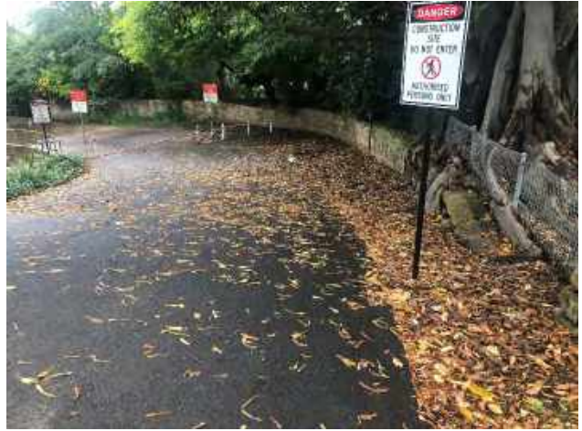
Plate 4.8. Driveway off Marsden Street, leading down to the weir, view facing southwest. Observations suggest a steeper natural slope than the path to the weir itself (Plate 2.2), suggesting more substantive earthworks at this location.
