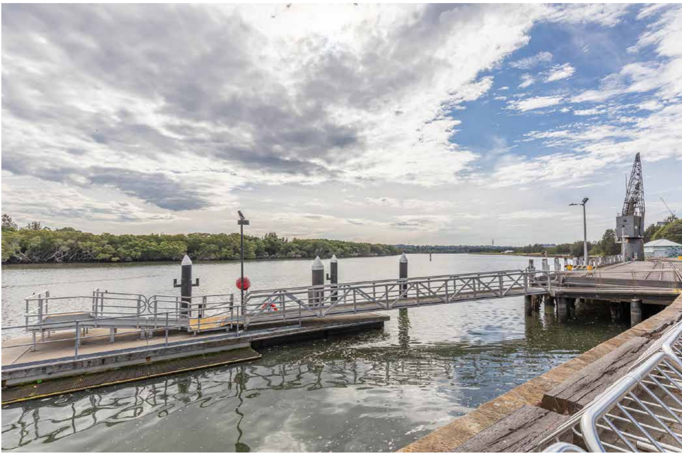
View 3 - Site from Armory Wharf
