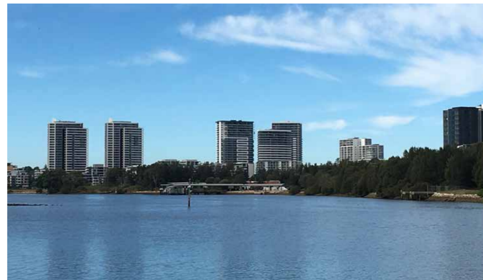
FIGURE 1.8. Rhodes precinct overlooking the Parramatta River
