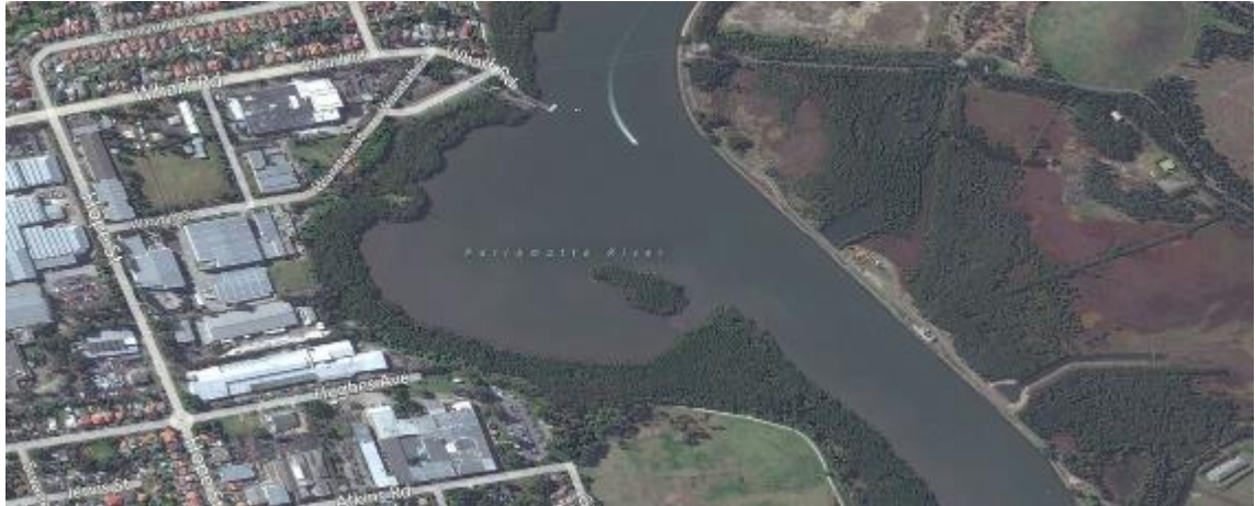
Figure 27: Site Analysis: Birds eye view of Wetlands within South Precinct and adjacent Parramatta River (Source: https://www.bing.com/maps )
