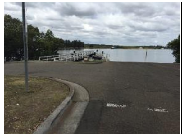
Fig. 29: Ermington Wharf (Heritage Item 82) – Wharf Rd
