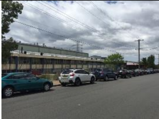
Fig. 54: Typical adjacent industrial
