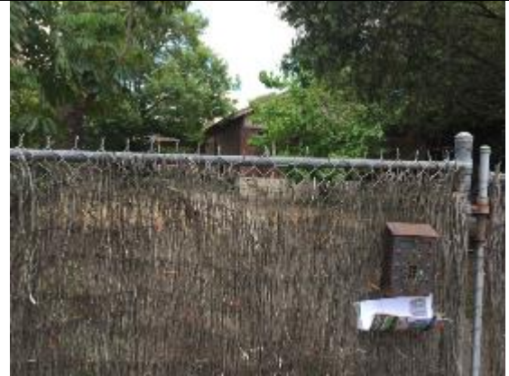
Fig. 45: Bulla Cream Dairy (Heritage Item 64) – Hughes Street
