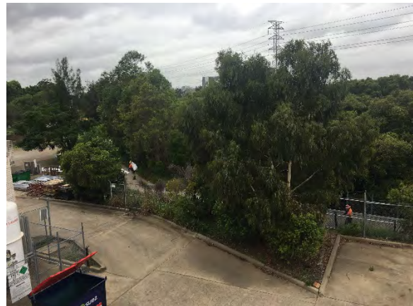
Photo 4. Looking towards the southern boundary of the site. A stormwater drain is visible along the southern fence line.
