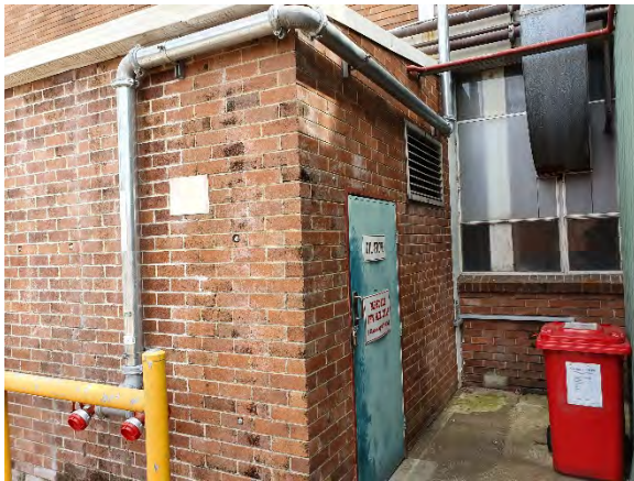
Photo 7. Oil store along the southern access road at the site.
