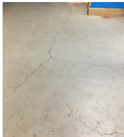
Photo 4. Cracking in floor of warehouse.
