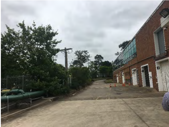
Photo 7. Western side of the property. Diesel storage for backup power generator located within building in this area.
