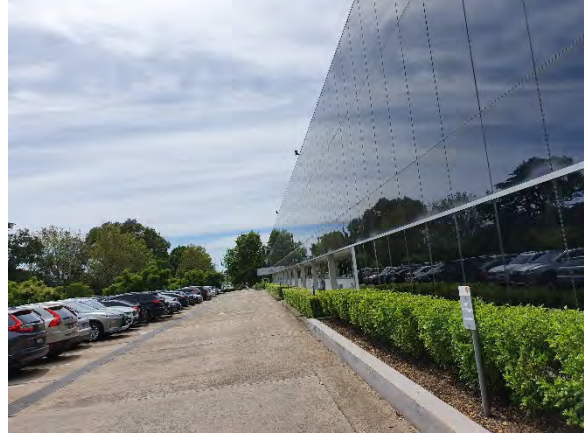
Photo 2. Administration building looking east.
