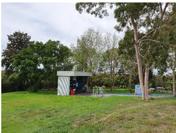
Photo 5. Drum store in the south eastern portion of the site.
