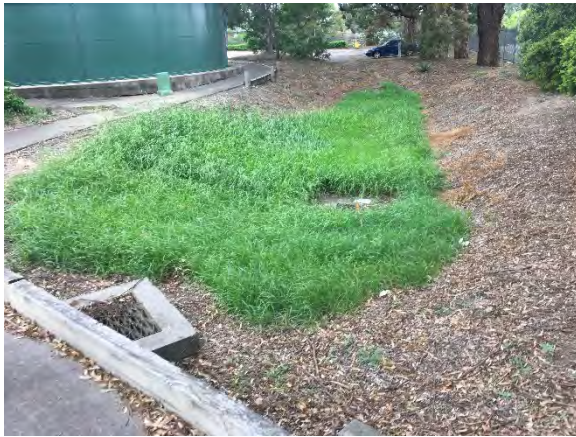
Photo 1. Stormwater retention basin.
