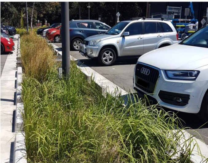
Swales in carparks or near other large areas of pavement collect stormwater runoff and remove pollutants
