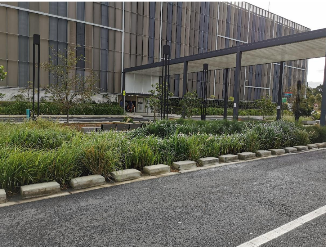
WSUD at Northern Beaches Hospital
