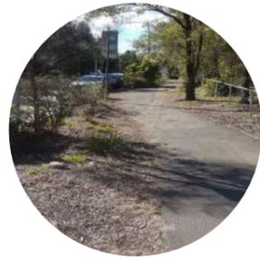
Poor condition of existing pedestrian asphalt path. Safety concerns due to vegetation and lack of lighting.
