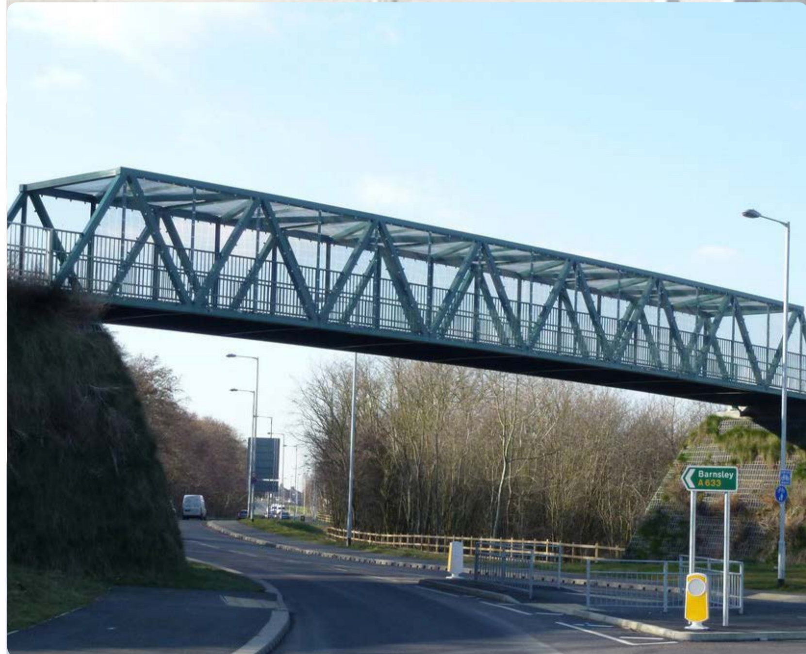
Hill Road Bridge will be either a 'through truss' (above image) or 'concrete beam' (below image) pending detailed design. Haslams Creek Bridge will be a 'through truss' (above image).
